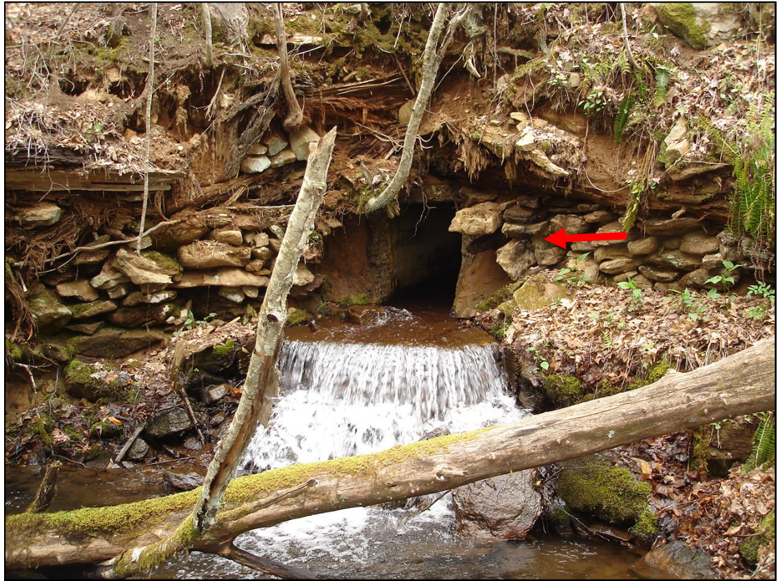
Plate 6 (below). Showing the spillway (red arrow) and downstream face of the dam in 2015. Note the amount of erosion that has taken place due to water topping the dam because of beaver activity.
