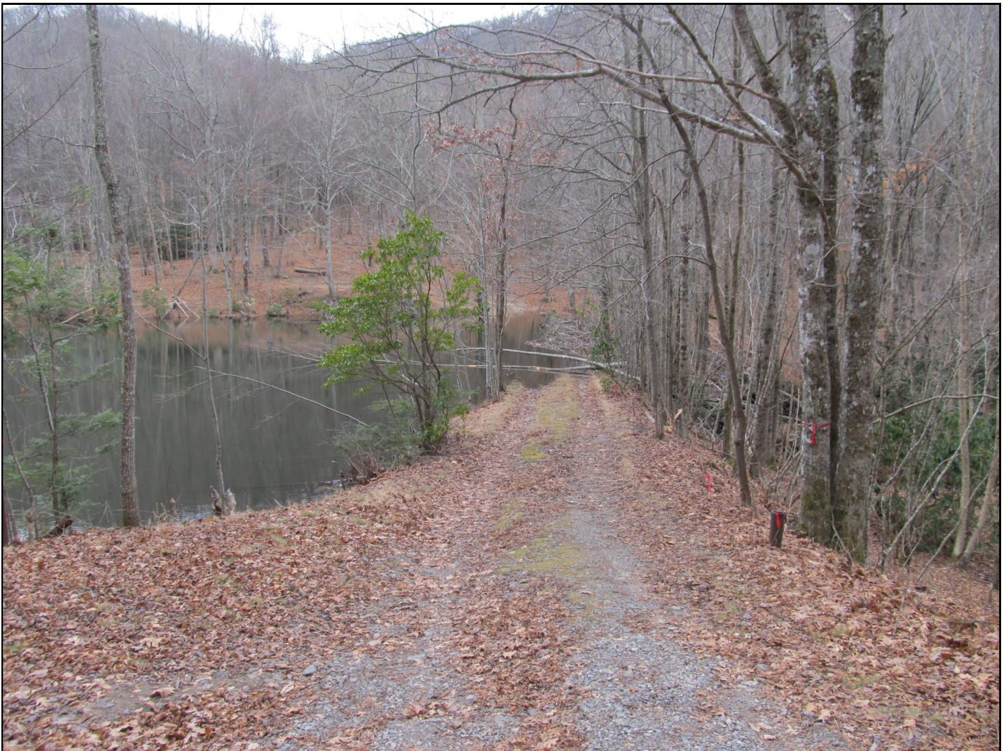
Plate 1. View south, showing the approximately 150 feet long, 18-foot tall earthen dam across Little Buck Creek. Photograph taken from FS Road 71. Note in the background that the water level is above the roadway across the dam due to beaver activity.
