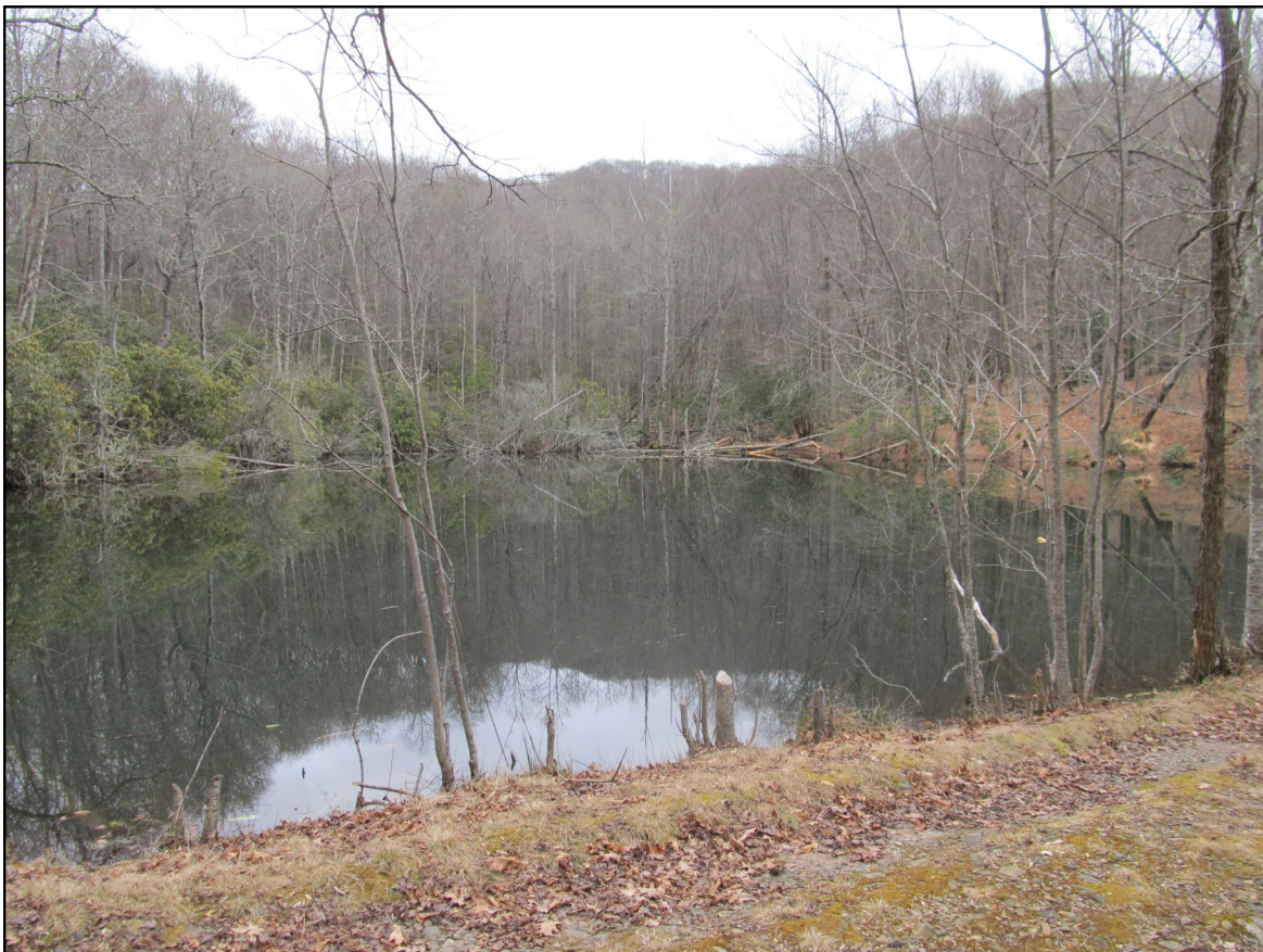
Plate 2 (top). Showing the 1 acre pond created by the Little Buck Creek dam.
